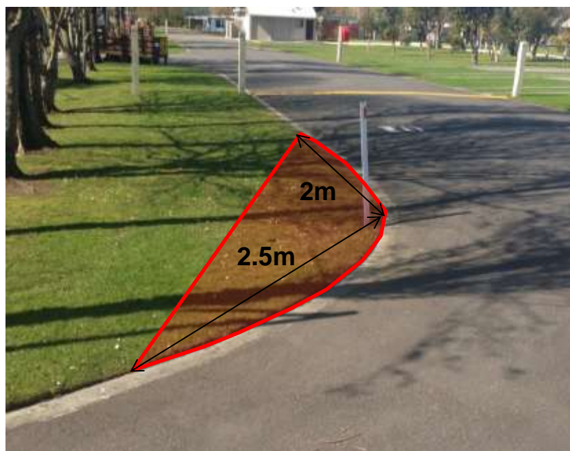
Figure 5.6: Intersection sight envelope to be kept clear of parked vehicles and objects that obstruct sight distances
